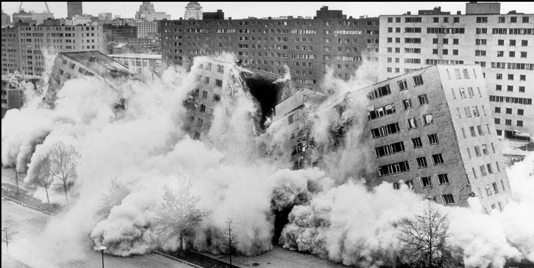
nationally televised demolition of a building of the pruit and igoe complexes , 1978
